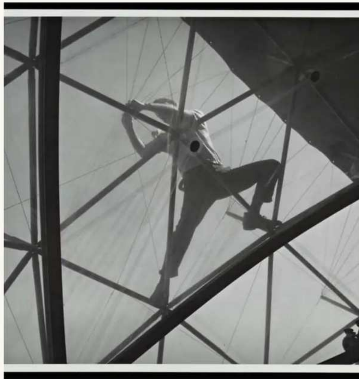
BERNARD JUDGE SPREAD ACROSS THE LATTICE, FIXING THE LINES THAT HOLD THE SKIN, SEEN FROM INSIDE. JULIUS SHULMAN, 1963, JOB 3378, FRAME 29; GETTY RESEARCH INSTITUTE. LICENCE REQUIRED.
