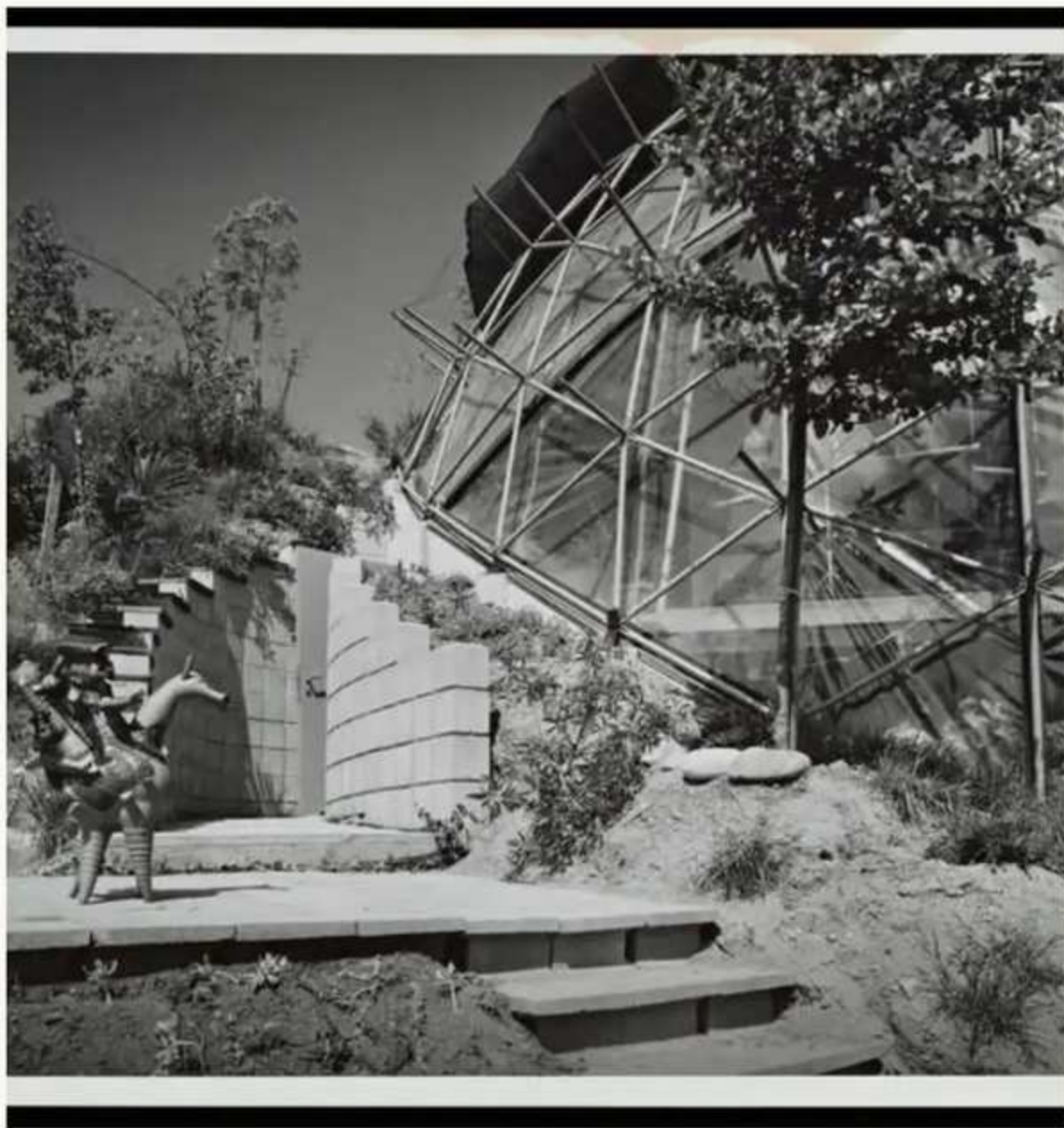
THE FRAME WITH THE SKIN PARTLY APPLIED, A FIGURE WITH A CAMERA ON THE STEPS OF THE CUT. JULIUS SHULMAN, JOB 3378, FRAME 3, 1961-62. DATE TO BE CONFIRMED; GETTY RESEARCH INSTITUTE. LICENCE REQUIRED.
