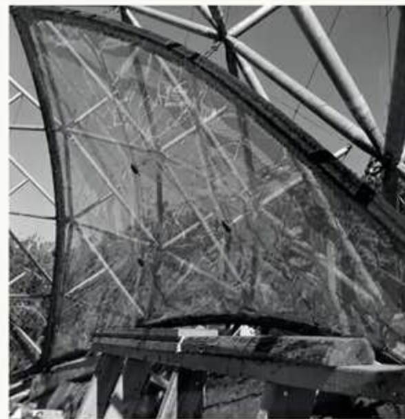
CLOCKWISE FROM TOP LEFT: THE CREW INSIDE THE FRAME, A GROUP PORTRAIT ON THE PLATFORM (READING-ROOM CAPTURE); FIGURES CLIMBING THE LATTICE, BENEATH A HUNG PANEL OF SKIN; THE FIRST PANELS OF SKIN STRETCHED OVER THE STRUTS, CLOSE; A MAN STANDING ON THE CROWN OF THE BARE FRAME, THE HILLS BEHIND. BLACK-AND-WHITE, 1958-61; THE THREE CONTACT-SHEET FRAMES ENHANCED (UPSCALED). JUDGE PAPERS, UCSB ADC 335; SCAN TO ORDER.
