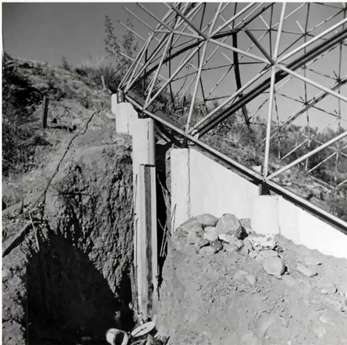
THE TRENCH AND THE BLOCK RETAINING WALL AT THE CUT. THE FRAME STANDING ABOVE. BLACK-AND-WHITE, UNDATED, 1958-59; ENHANCED (UPSCALED) FROM THE JUDGE PAPERS FRAME. UCSB ADC 335; SCAN TO ORDER.
