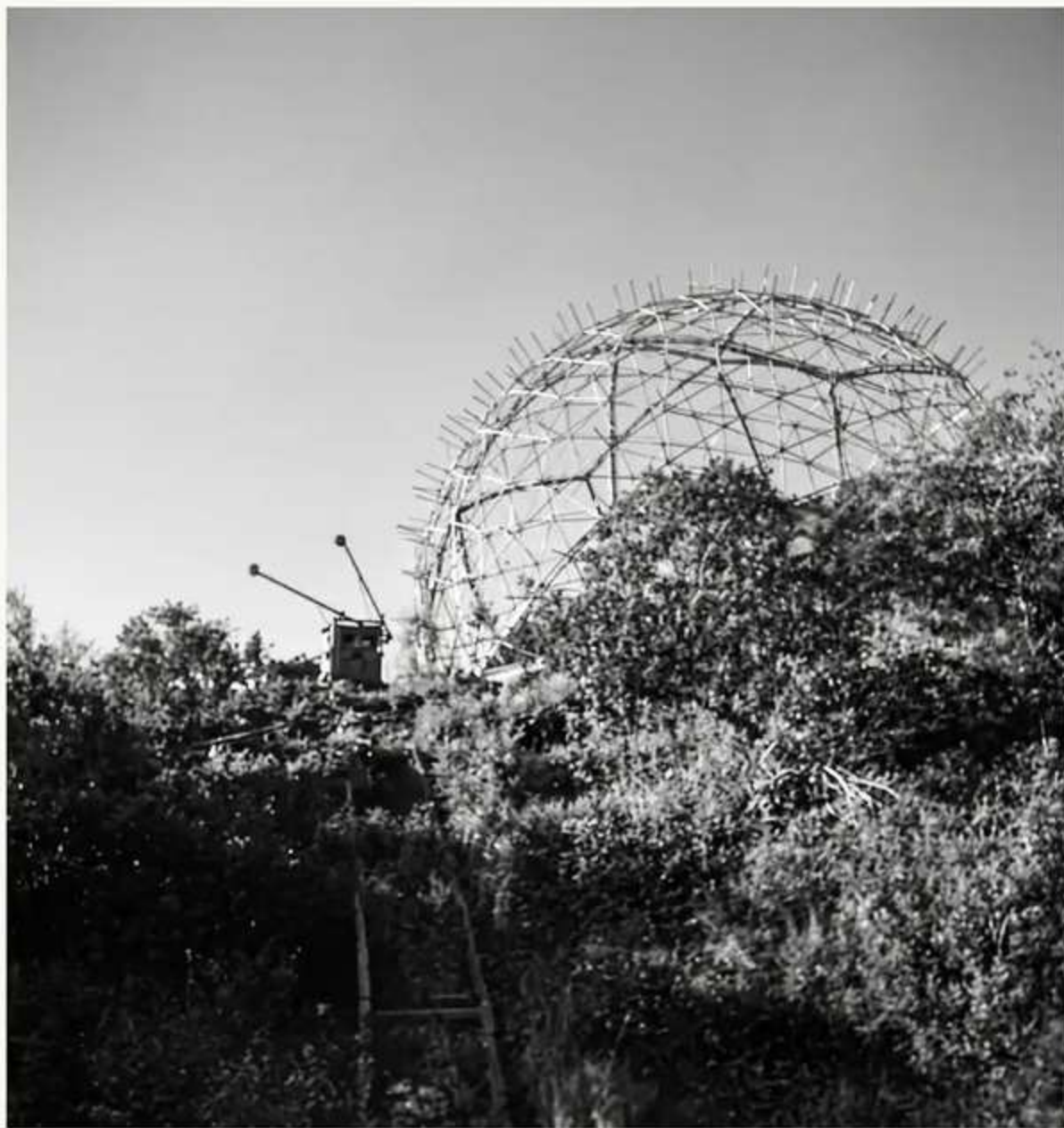
THE BARE FRAME ON ITS RIDGE SEEN FROM THE CANYON BELOW, THE TRIPOD HOIST RESIDE IT. ENHANCED (UPSCALED) FROM THE JUDGE PAPERS FRAME. UCSB ADC 335; SCAN TO ORDER.
