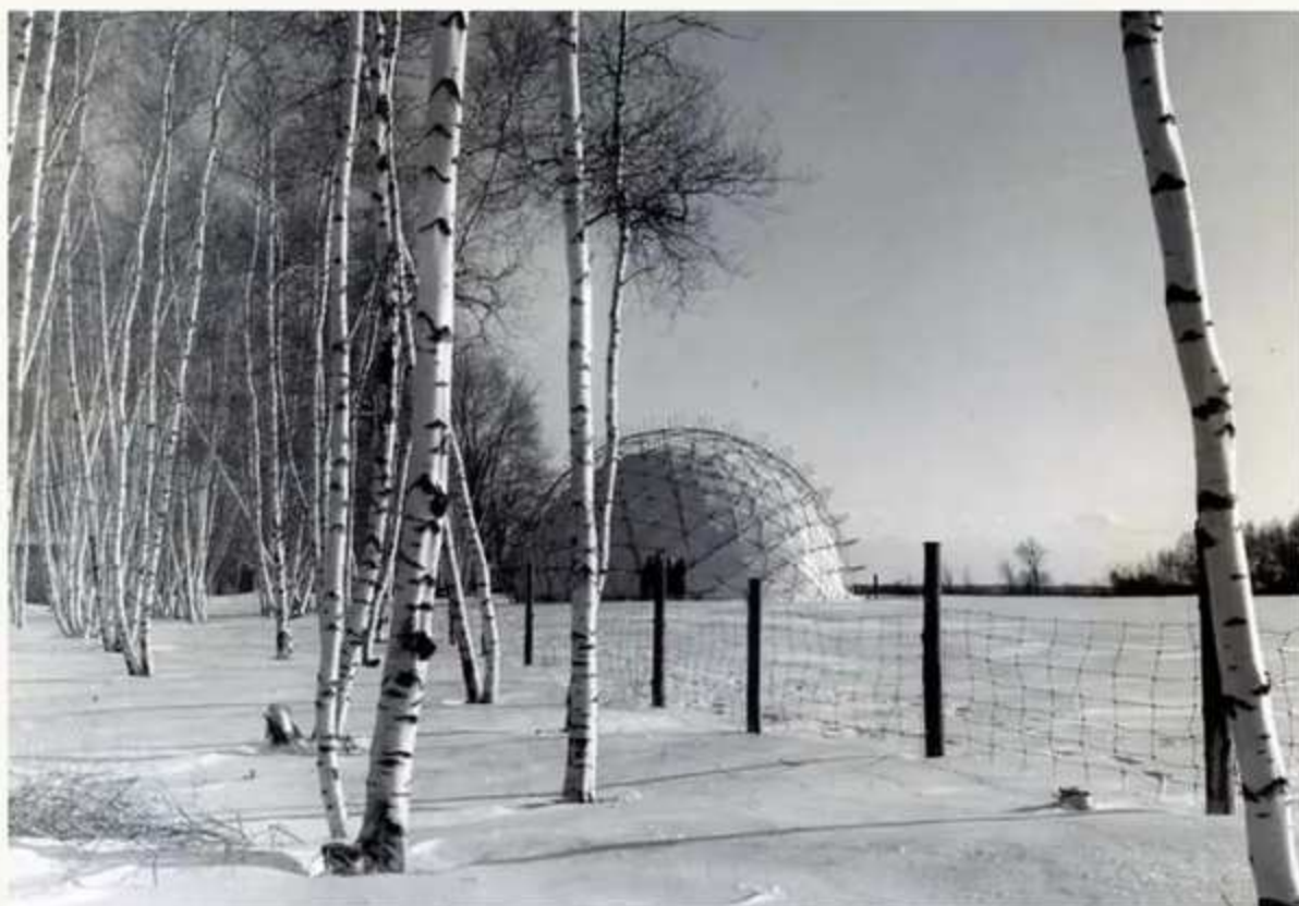
WEATHERBREAK FROM THE ROAD THROUGH THE BIRCHES, BAIE-D'URFÉ, DECEMBER 1950. FORDS JEFFREY LINDSAY, CANADIAN ARCHITECTURAL ARCHIVES, UNIVERSITY OF CALGARY.
